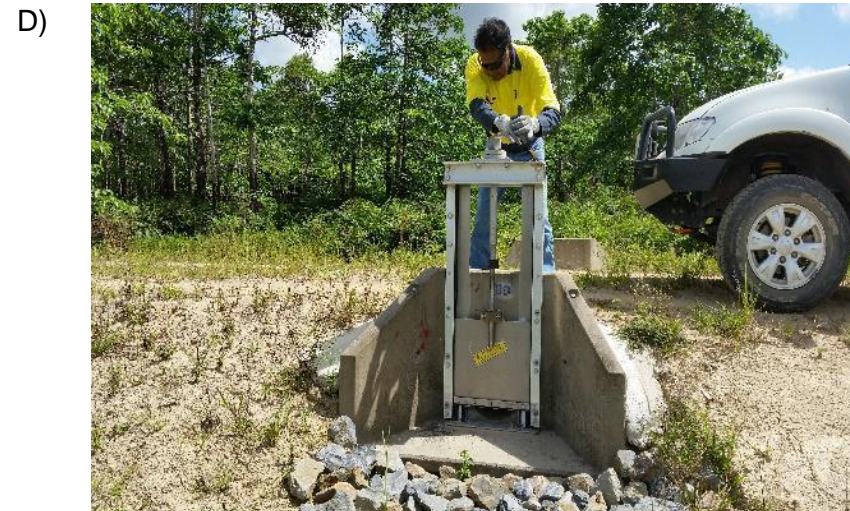
Figure 6: Babinda constructed wetland showing location of the inlet control structure between the wetland and the Babinda drain, position of the diver loggers (Logger 1, Logger 2) recording water depth, water temperature and conductivity, the outlet weir, and the twelve manually control outlet pipes
